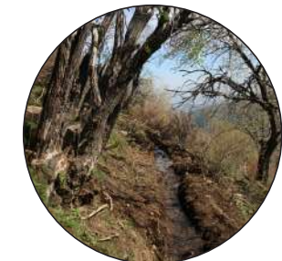
Most of the channels are hand-made using stones and mud collected in site. This way of construction makes them partially permeable to water, allowing leaking and watering of downhill pastures. ©LD
